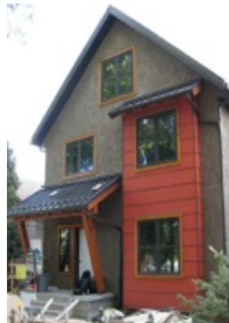
Mill Creek NetZero
