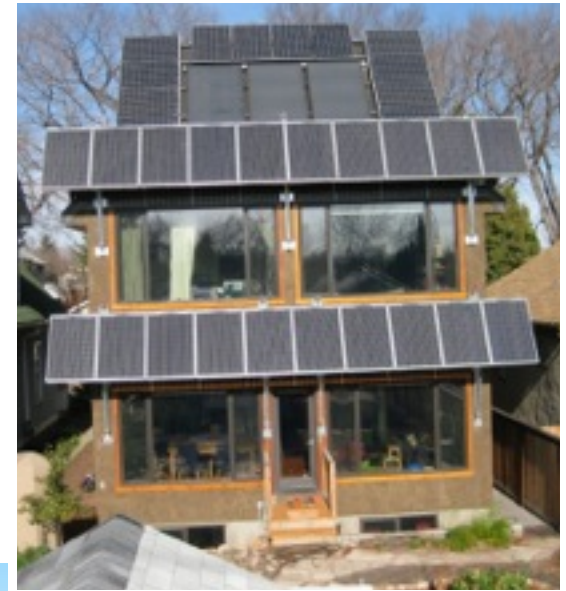
Mill Creek NetZero
